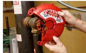
At this point, it's time to shut down the machine or equipment that will be serviced or maintained.
